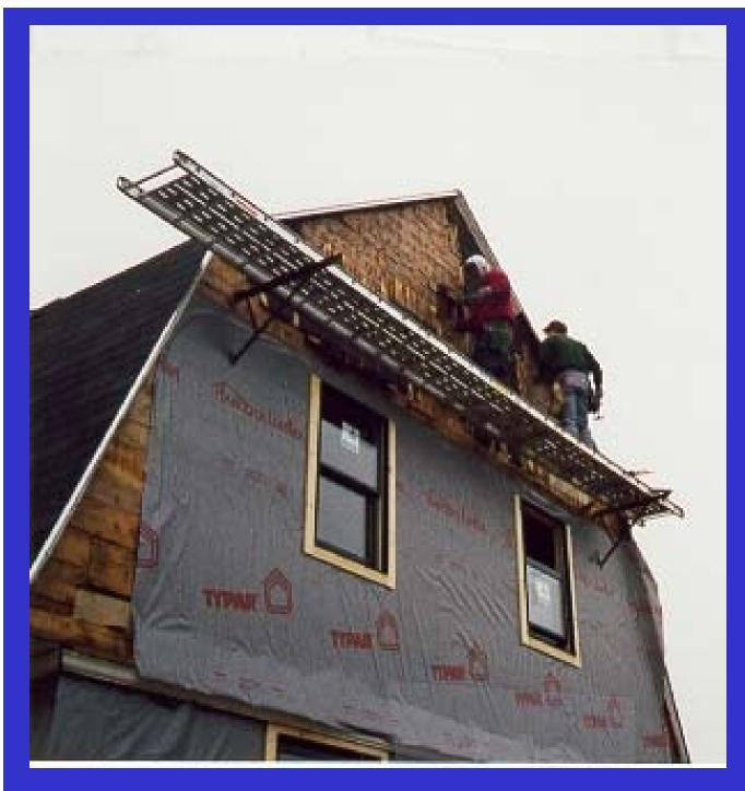
Again, there is no protective system installed. The workers could have used a harness or guardrail system along with end rails.
