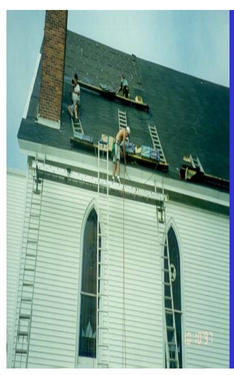
In a situation like this, full body harnesses with lanyards and/or a catch platform would be a suitable means of fall protection.
