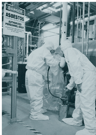
Asbestos removal
