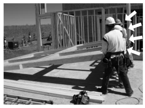
Good Practice: Manually raising balloon walls. Always calculate the weight of the wall to ensure you have enough employees to raise it safely. For example, a 9' x 15' wall with two 3' windows made from 2" x 4"s weighs 465 lbs.
