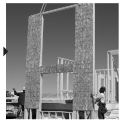
Best Practice: Use a crane. Booming walls using a crane is safer, faster, and uses less labor than manually raising walls.
