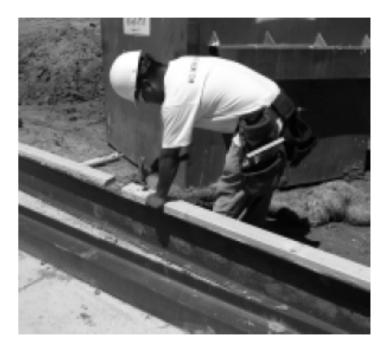
Attach your top plate before setting steel. You'll reduce your risk of a fall by not performing the task on a ladder and you'll eliminate working above shoulder height.
