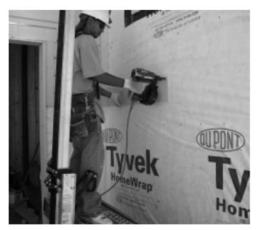
Keep the siding installation between waist and mid-chest height by making regular adjustments to the scaffolding plank height.
