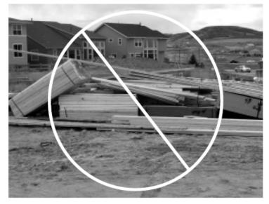
Avoid moving materials twice. Don't allow suppliers to drop off materials away from the foundation or stacked on top of each other. Materials dropped off next to foundation
