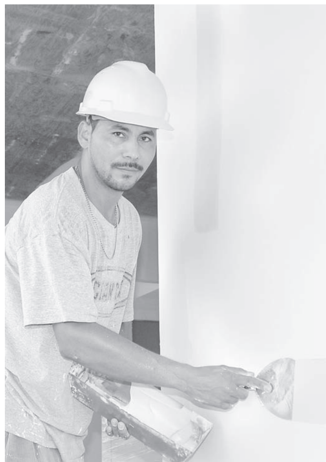
After the drywall is installed, tapers fill joints between panels with a joint compound.
