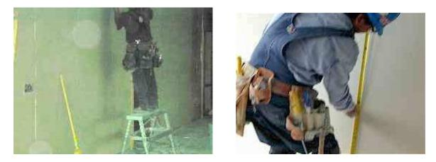
**Figure 5a, 5b.** Rotation from screw gun use (left) to other installation tasks (e.g., measuring/marking (right), cutting and installing panels.
