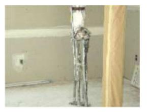
**Figure 9.** Stilts use – prolonged use can be stressful to legs, back.
