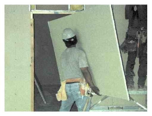
Figure 1. Lifting heavy wallboard panels for installation.
