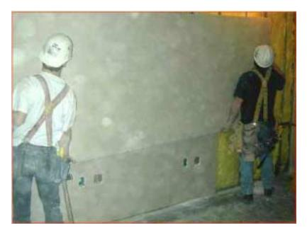
Figure 2. Two-worker panel lifting.
